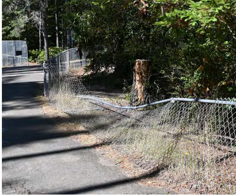
Fencing around the pond is failing. Estimated cost.....$50,000-85,000 » Reconstruct the fence, realignment.
