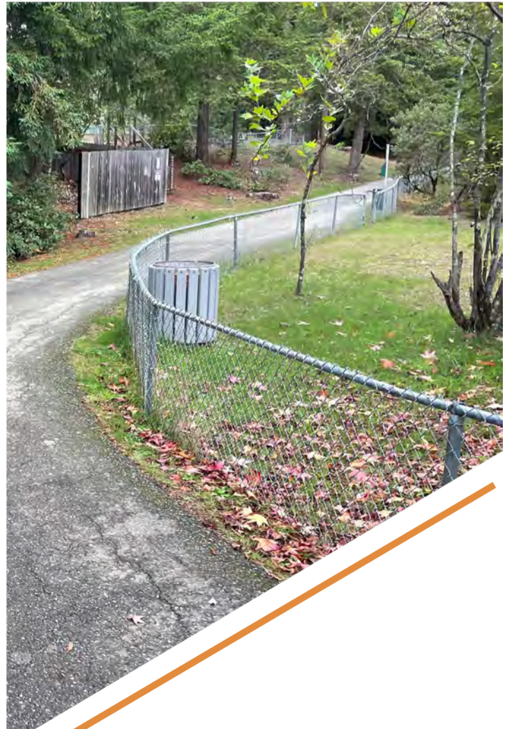
Fencing around the pond is failing. Estimated cost.....$50,000-85,000 » Reconstruct the fence, realignment.
