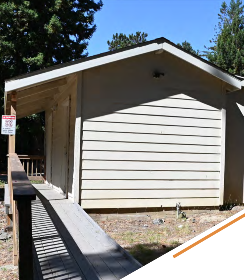
The transition from walkway to access ramp is not ADA compliant. There is no ADA parking near the restroom building. Estimated cost. .... $20,000-50,000 » Restroom upgrades, ADA ramp, lighting.
